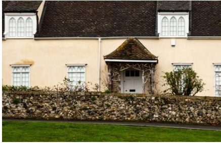
Examples of flint wall, white brick retention wall.
