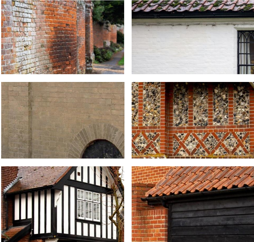
Examples of façade materials such as: red, white and yellow brick, timber frame, flint panel and black weatherboard.
