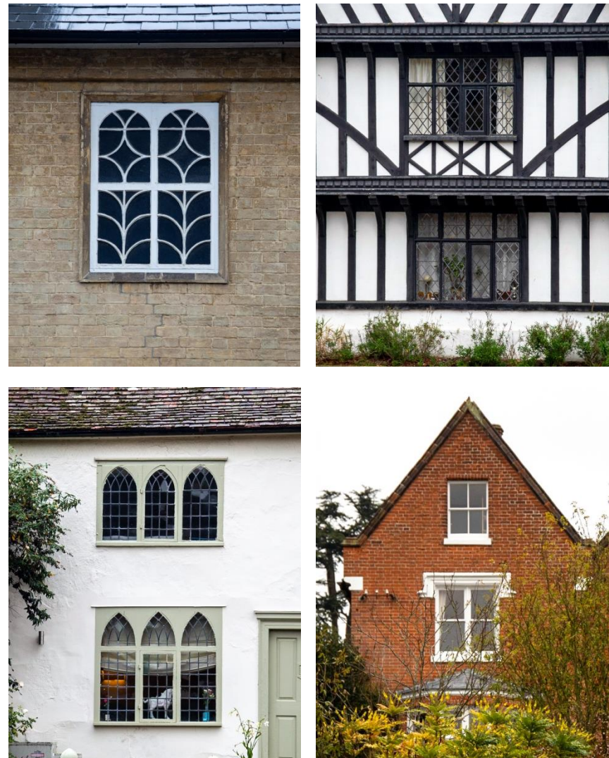
Examples of window detailing including gothic arch and Victorian paned timber.
