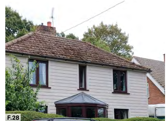
Figure 28: Photo of a dwelling with off-white weatherboarding and brown detailing.
