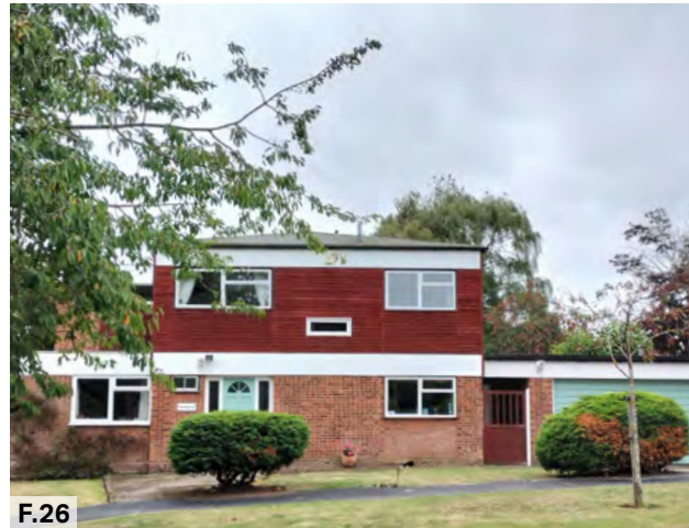
Figure 26: Photo of a dwelling with a mixture of red-brown weatherboarding, red bricks and white render.
