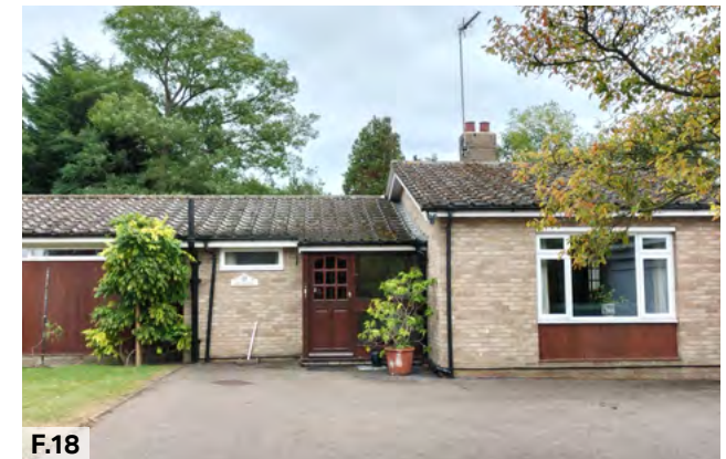
Figure 18: Photo of a more recent single storey development in Playford.
