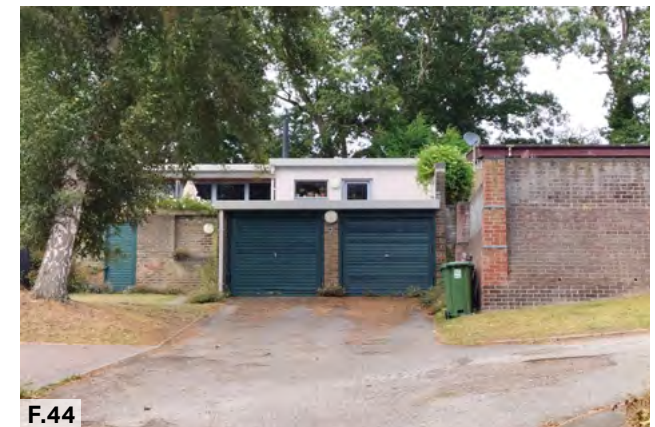
Figure 44: Example of on-plot garage parking in Playford.
