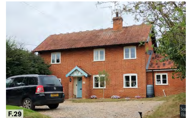
Figure 29: Photo of a dwelling with a red brick facade and matching extension, as well as a light blue front porch canopy.
