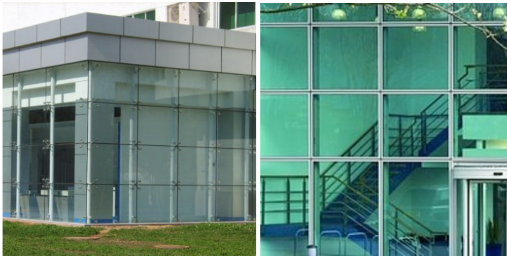
Figure 6. Framed and Frameless Glass Curtain Walls
