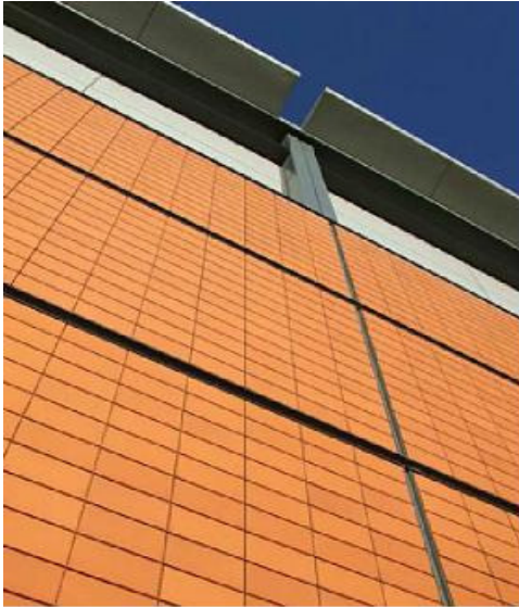
Figure 3. Terracotta rain screen cladding
